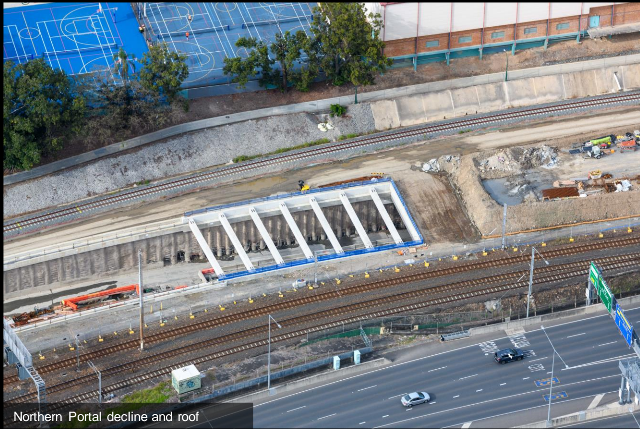
FRP and concrete works ongoing beneath portal roof
