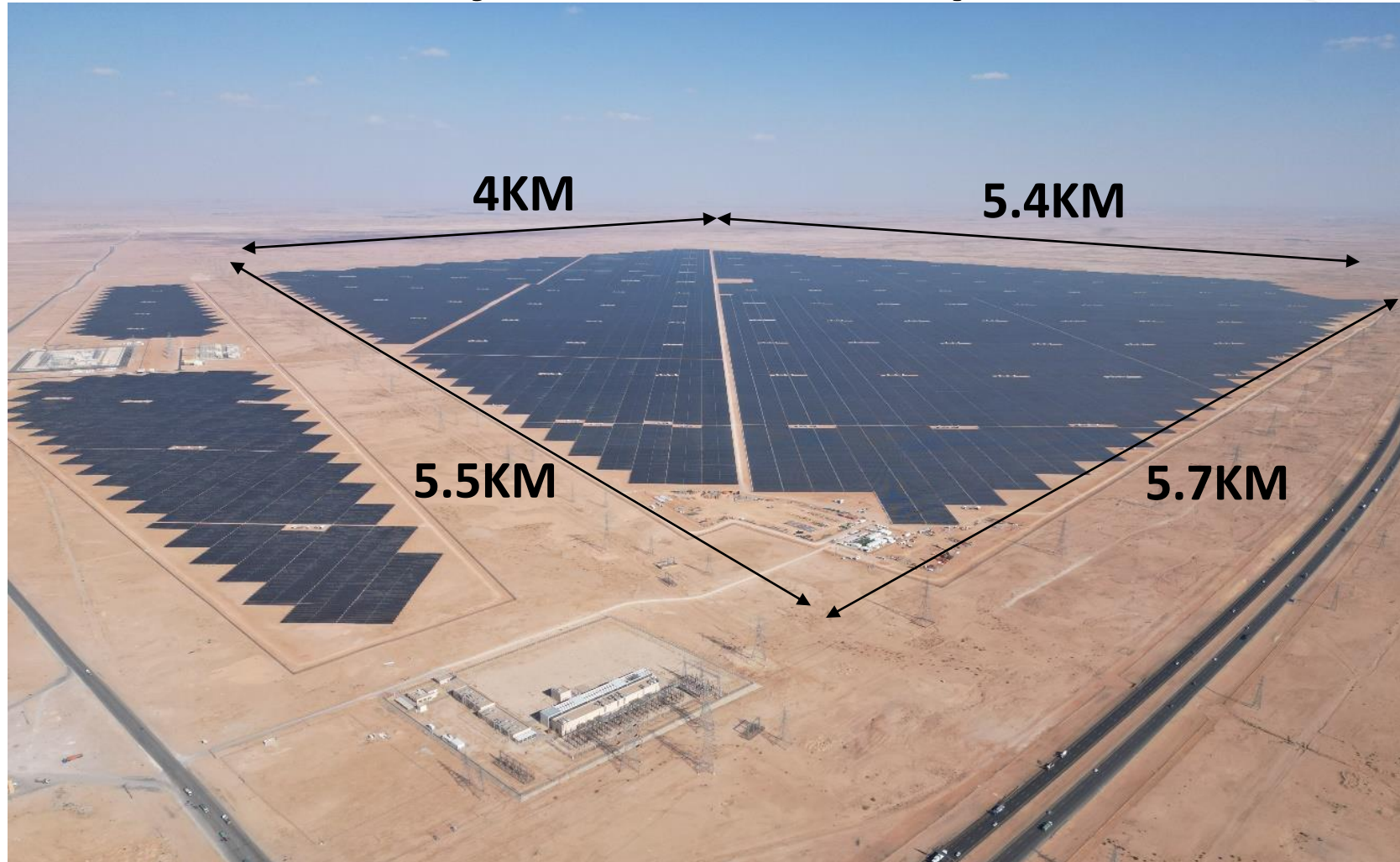
Complete PV Plant, (Sudair PV Plant, KSA, 1500MW)
