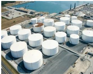
Hydrocarbon Storage Tanks
