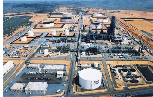
Crude Oil Processing and Desalination Units
