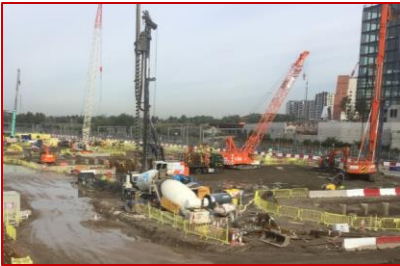
Stratford Waterfront Construction Starts
