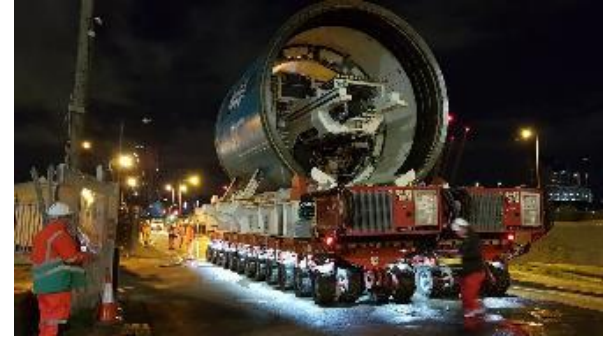
Greenwich TBM delivery utility issues
