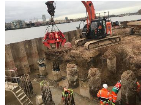
King Edward Memorial Park Foreshore Cofferdam Stability
