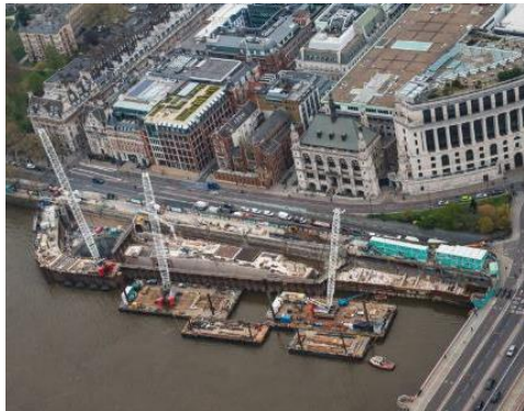
Blackfriars Gas Main Utility Diversion
