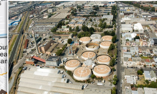
Southeast Treatment Plant
