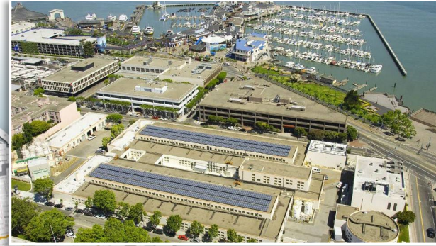
North Point Wet Weather Facility
