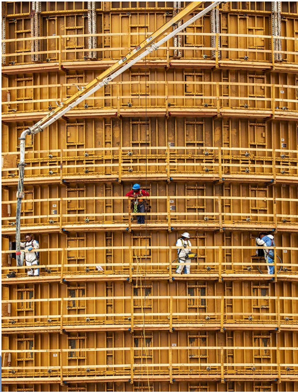
June 7, 2023: Biosolids Digester Facilities Project: First digester core wall pour.
