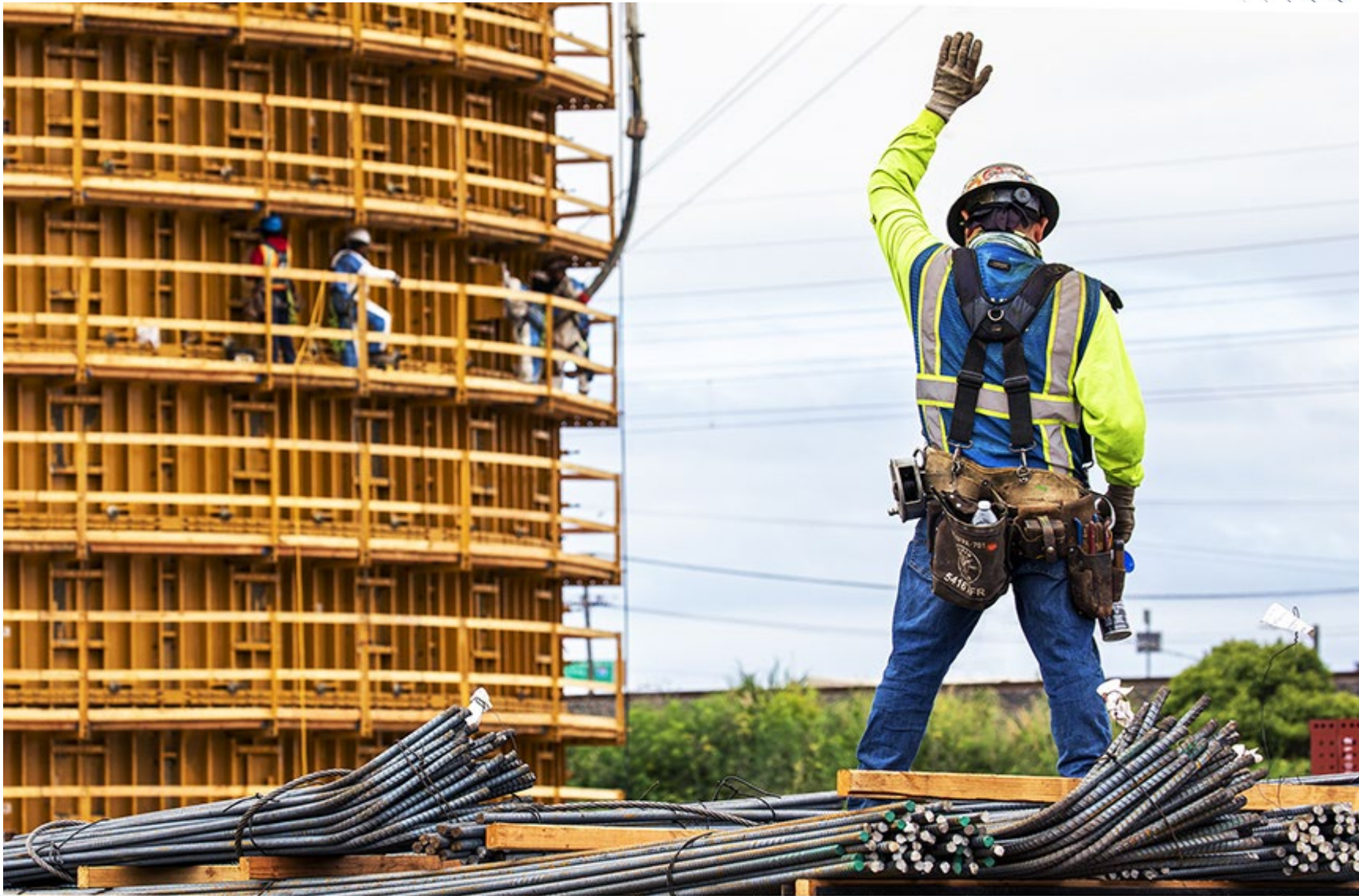
June 7, 2023: Biosolids Digester Facilities Project: First digester core wall pour. Worker signaling to crane operator -rebar lift.
